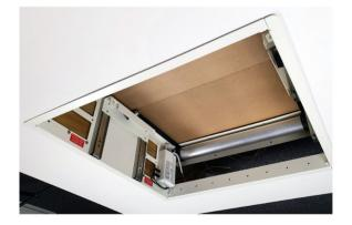
4. Wire power into the lift and bring the lift to the lower position using the manual buttons on the control box. You may need to pull down on the slider mechanisims as they do not have the weight of the projector to move them. Connect the required 12volt trigger cables and test the remote operation of the lift and screen. This can be done with a 9v PP3 battery. Bring through the AV cables from the rear of the lift.
